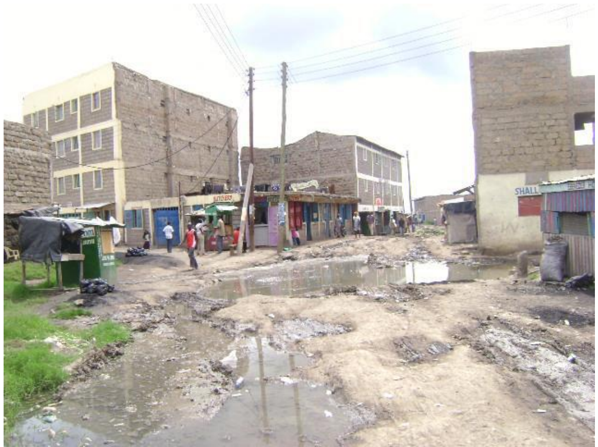
Open discharge of raw sewage in drainage channel along a road (Source: Field survey)
